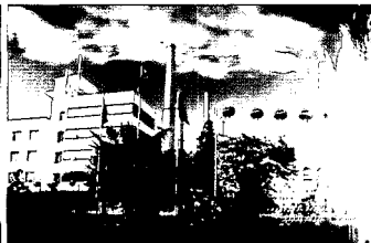
Dou He Power Plant
