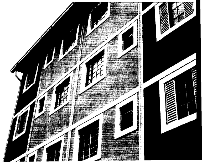
Housing project erected with Usiteto technology in Timóteo, MG
