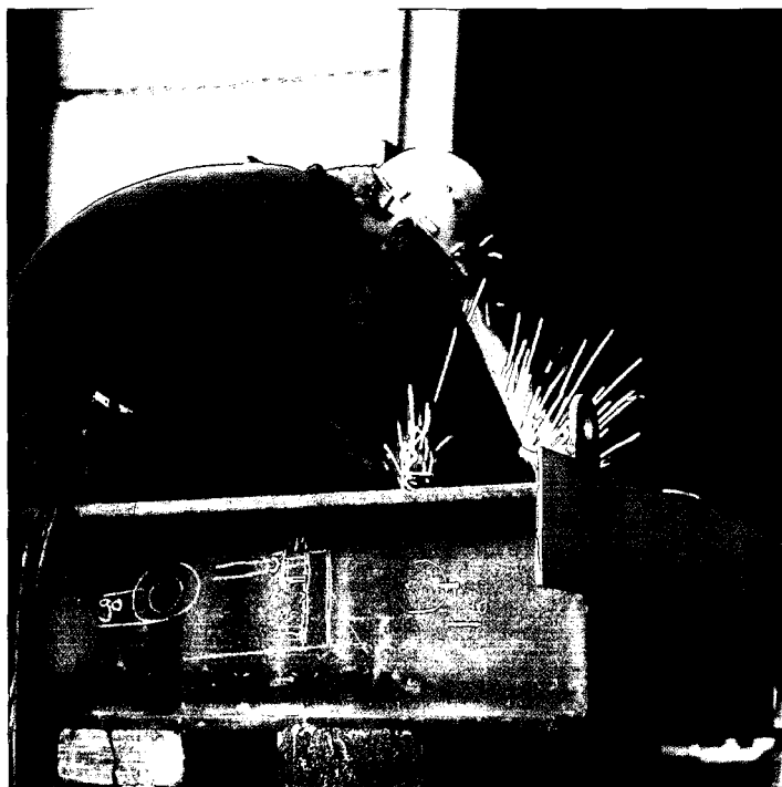
Welder doing construction work at the IHC Merwede shipyard in Sliedrecht, The Netherlands.
