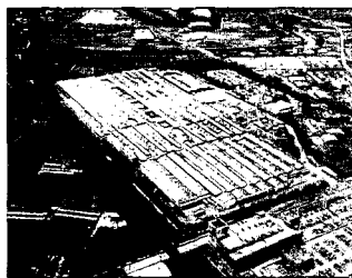
We are concentrating our Japanese tire production on high-value-added products. The Tosu Plant, shown here, was the first plant in the Bridgestone Group to mass-produce runflat tires.
