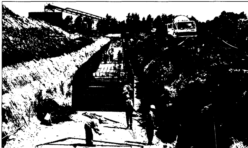
Construction of the Leeuwan jig plant which will enable production of a further 1Mtpa of power station coal.
