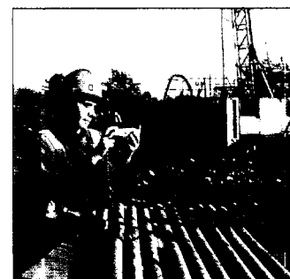
Nickel Rim South nickel project, Sudbury – shaft sinking will be initiated in 2005 along with further underground development drilling.
