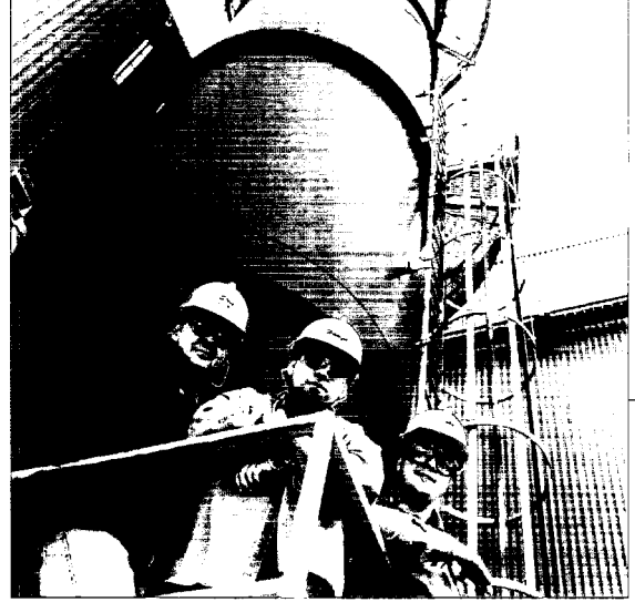
Steve Adams, Hamza Al-Habbal and John Lundrigan at the new odour neutralizing and reducing equipment at Dofasco's Continuous Pickling Cold Mill (CPCM).
