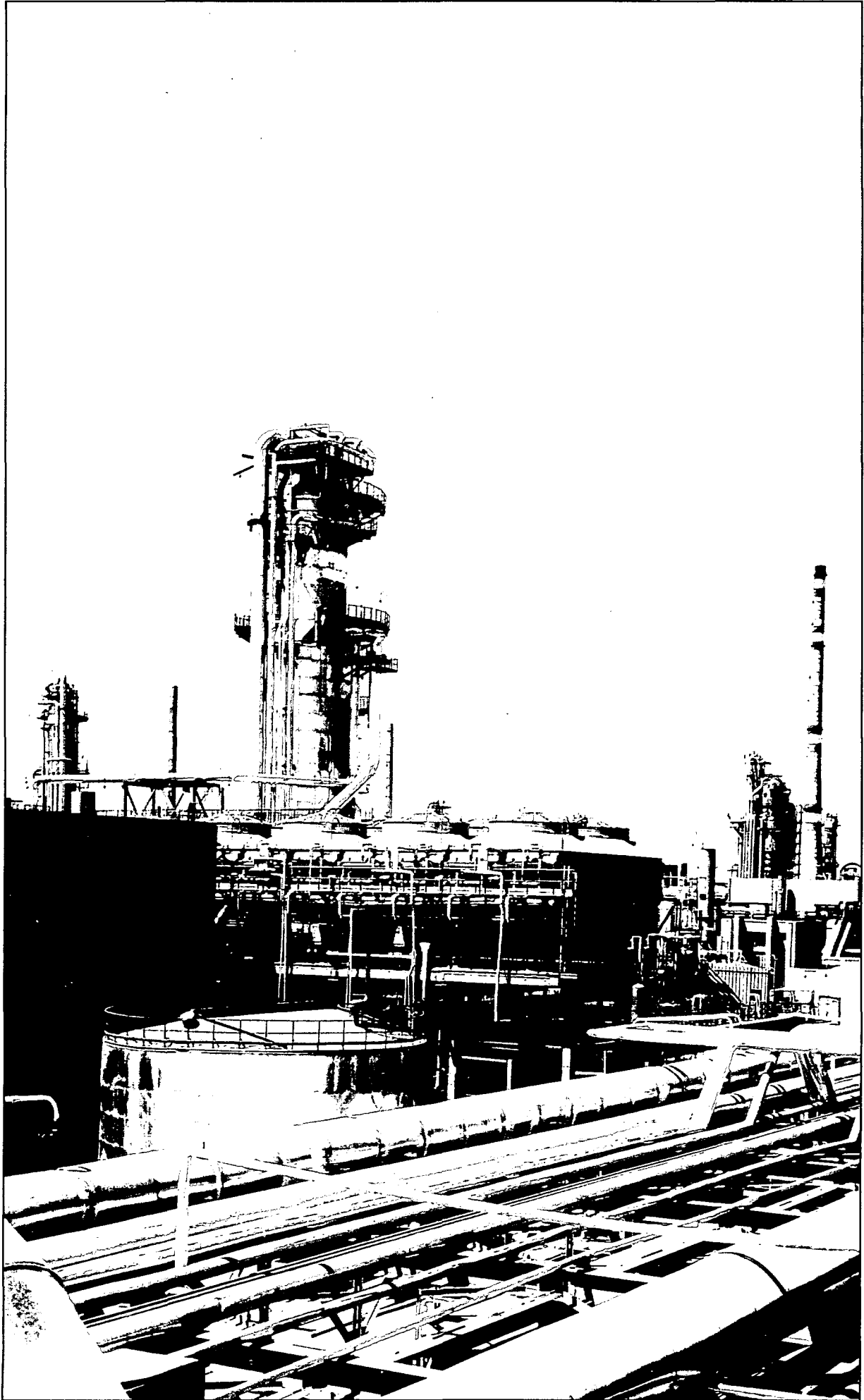
Gas Processing Plant
