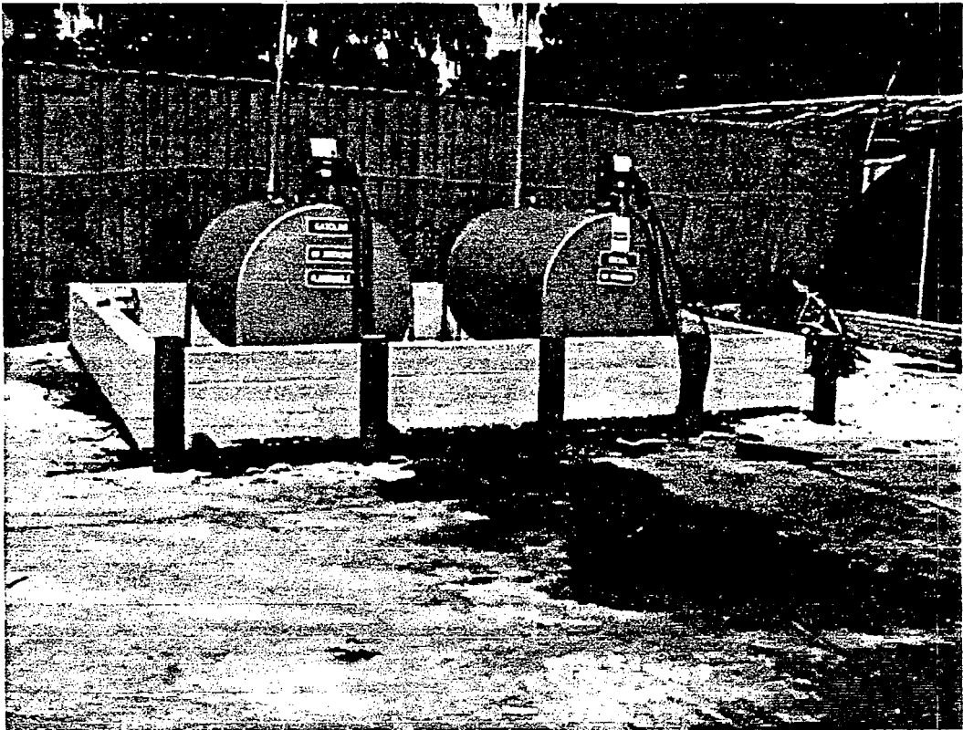
Above Ground Storage Tanks at Maintenance Facilities
