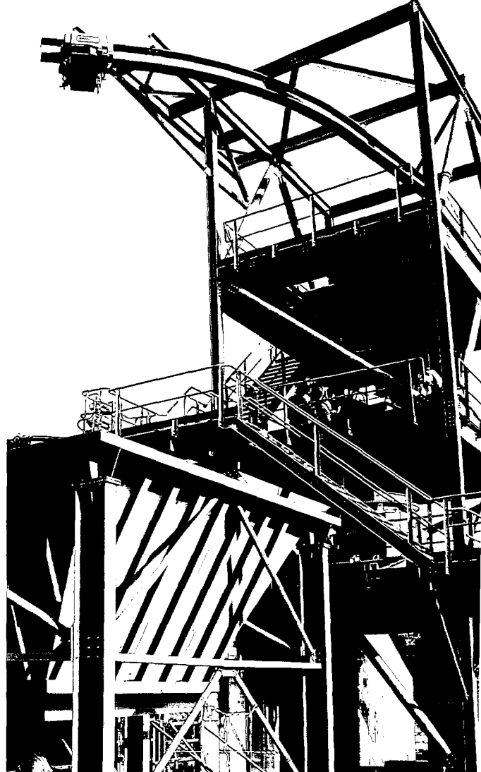
Aguablanca Construction Activity in 2004
