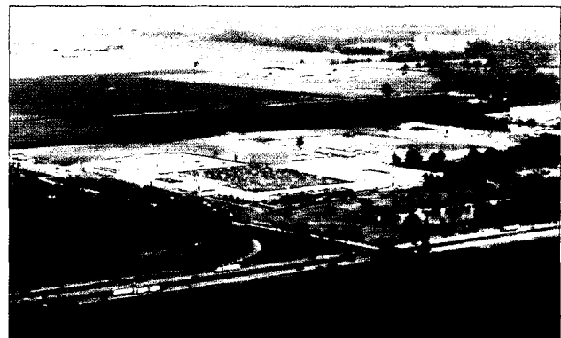
TIEM's plant in Columbus, Indiana
