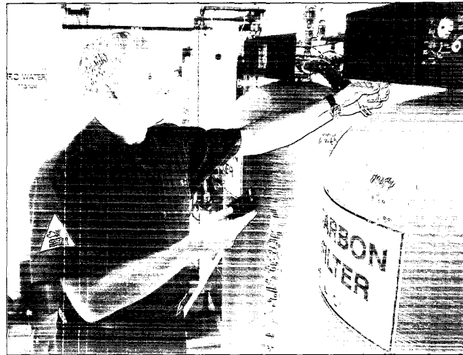
Ultra-pure Water Treatment System for Dialysis Clinic
