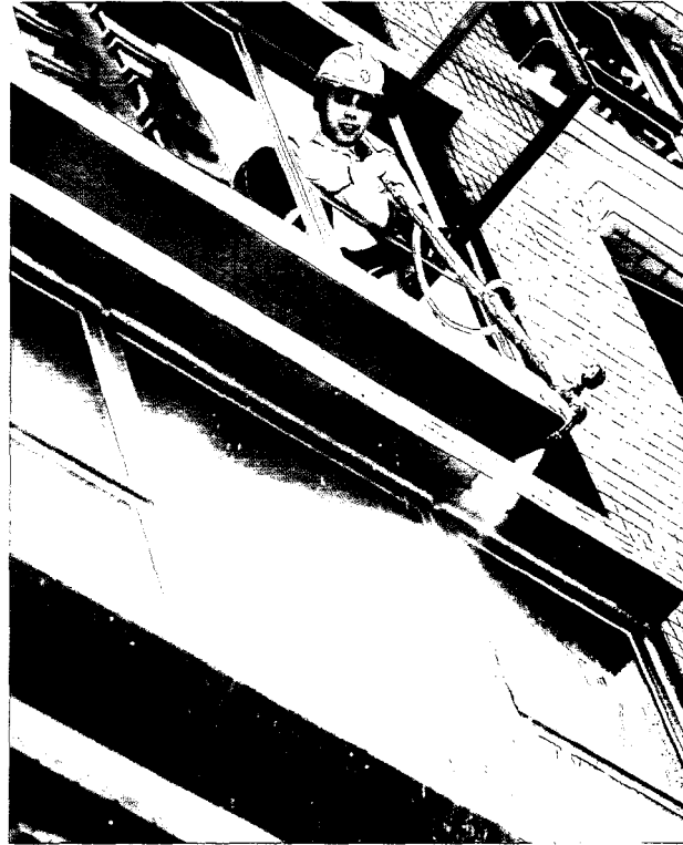
The Group tests every window in new developments with a high-pressure water spray after installation.
