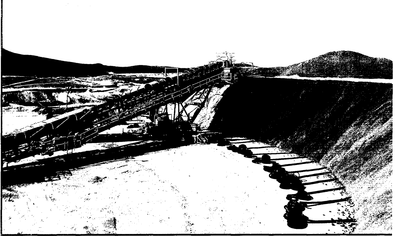
Stacking ore on leach pads at Quebrada Blanca
