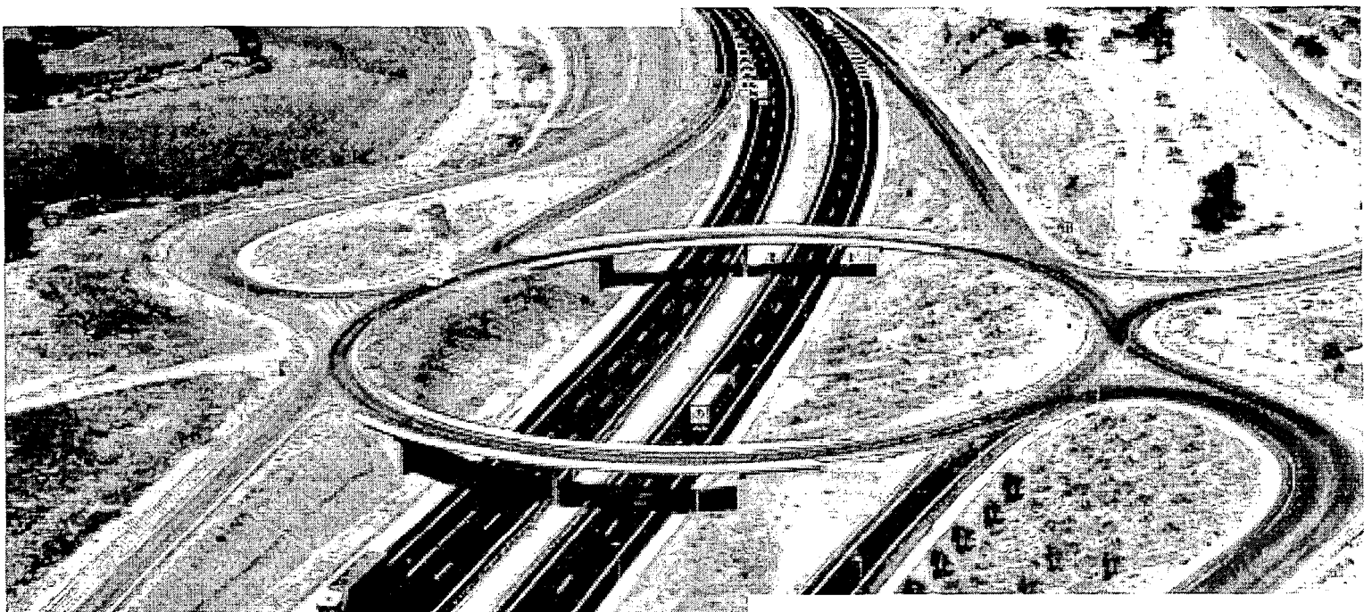
Lleida-Barcelona Divided Highway. Section: Santa Maria del Cami-Igualada (Barcelona). Elevated traffic circle.
