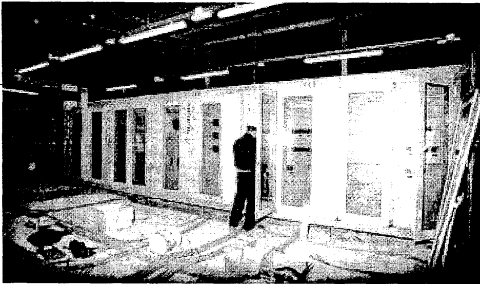
Electrical installations at the Sogecable building, Madrid.
