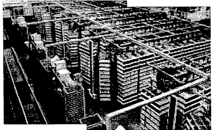
Automatic picking installations.
