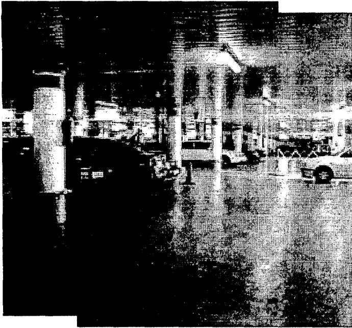
Underground parking in Granollers (Barcelona).
