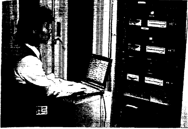
Maintenance work of servers with the use of FST
