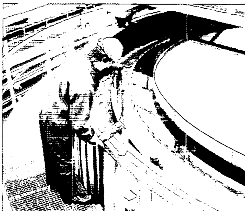
ONE OF OUR ENVIRONMENTAL INVESTMENTS IMPLEMENTED DURING 1997 - WASTE WATER (TREATMENT) SYSTEM IN DUNA REFINERY
