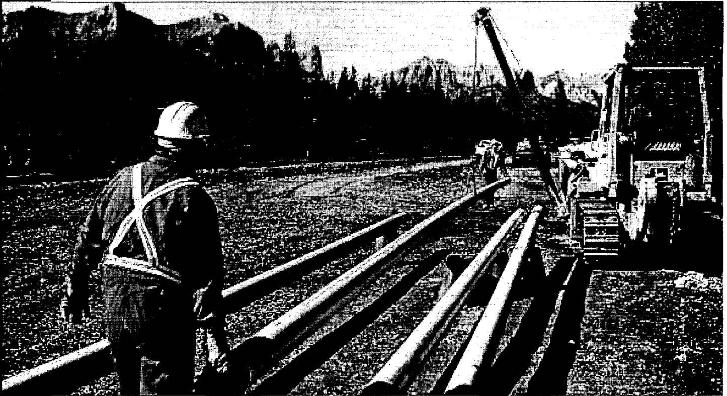
ATCO Pipeline installation near Exshaw, Alberta
