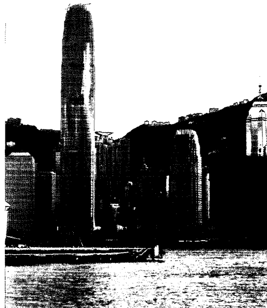
Supply and Installation of ELV Systems includes Digital CCTV Surveillance Systems, Security System, Giga-bit Ethernet fibre backbone, SMATV, Walkie Talkie, Radio Paging System and Public Address System at Two International Finance Center, the 88-storey class A intelligent commercial building at Central
