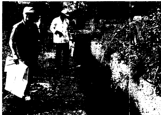
BANAN – TRENCH TRENCHING OPERATIONS IN BANANKORO
