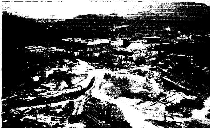
Tai Po Water Treatment Works and Pumping Station for Water Supplies
