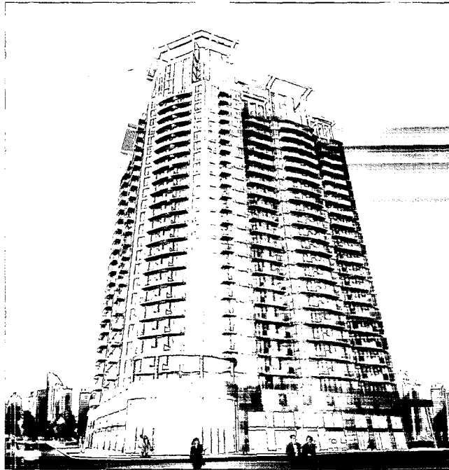
Chevalier Place, a first class residential project in Shanghai, was completed in December 1999
