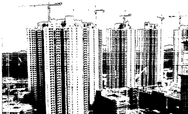
Public Housing Estate at Tin Shui Wai Area 105, Phase 1
