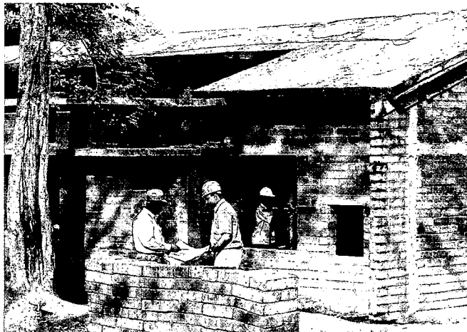
ITC's paperboard Unit uses fly ash waste from the factory to make bricks for constructing houses and roads.
