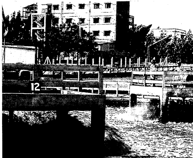
The effluent treatment plant at the Bhadrachalam Unit.
