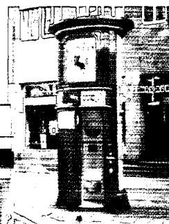
Column with integrated public toilet.
