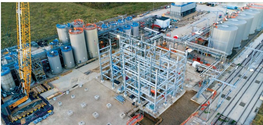
Construction in Progress: Alkoxylation Plant, Pasadena, Texas
