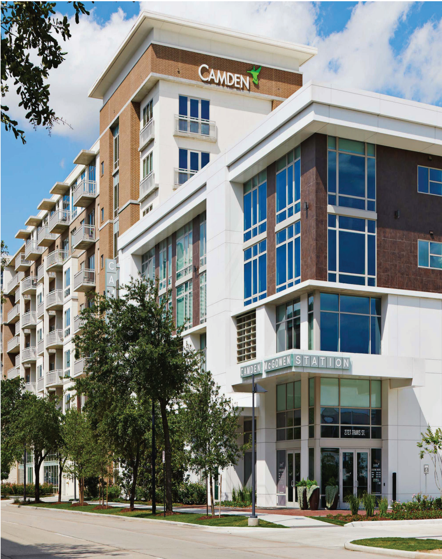
Camden McGowen Station, Houston, TX
