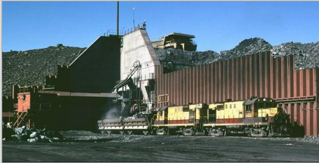
Figure 18-1: LTVSMC Rail Transfer Hopper in Operation
