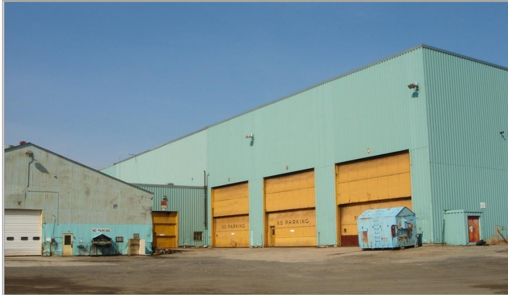
Figure 18-2: Area 1 Truck Shop viewed from the southeast showing the tracked equipment bays and tyre shop
