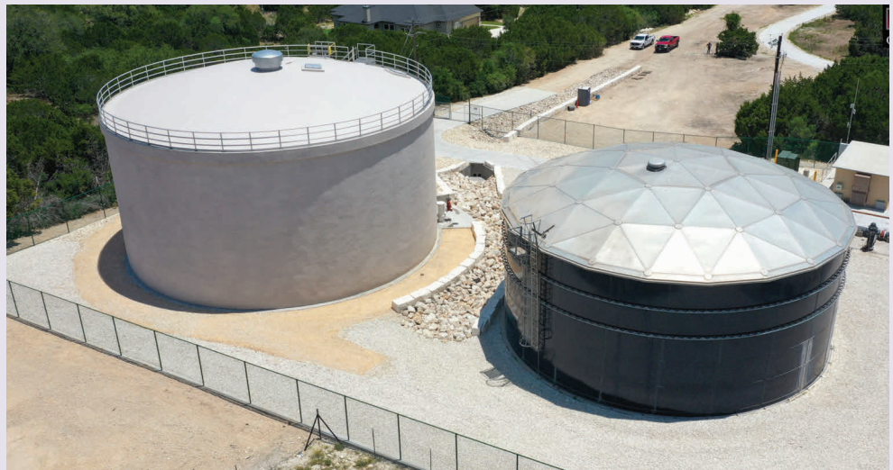
Comal County, TX — 750,000-gallon water storage tank completed at a cost of $2.2 million. One of 13 water storage projects completed, under construction, or in design.
