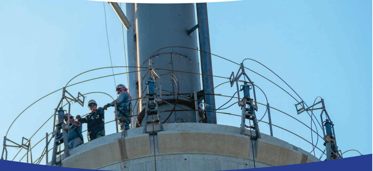
TWC's Alnwick water storage tank under construction.
