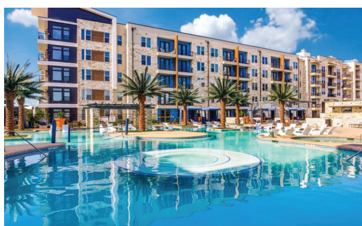
Vitruvian West Phase 2, Dallas, TX
