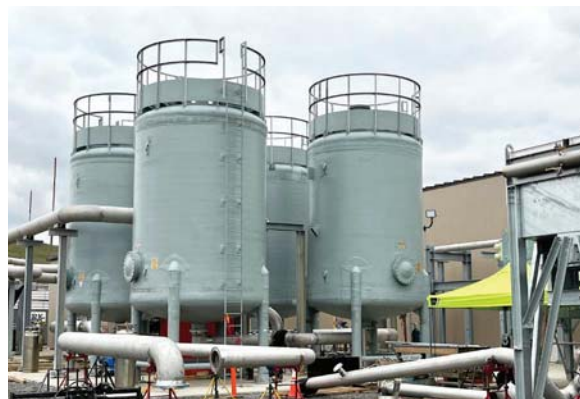
Construction in progress at the two RNG facilities EDL is building.
