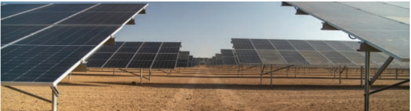
(Left to right) Female employees in the Women's Lounge at Tasiast. Kinross Chile participants in Kinross' bespoke safety excellence program, which has been completed by all sites. (Above) Tasiast solar plant, which includes approximately 78,000 panels, 34 MW capacity (Alternating Current) and 18 MW of battery storage.
