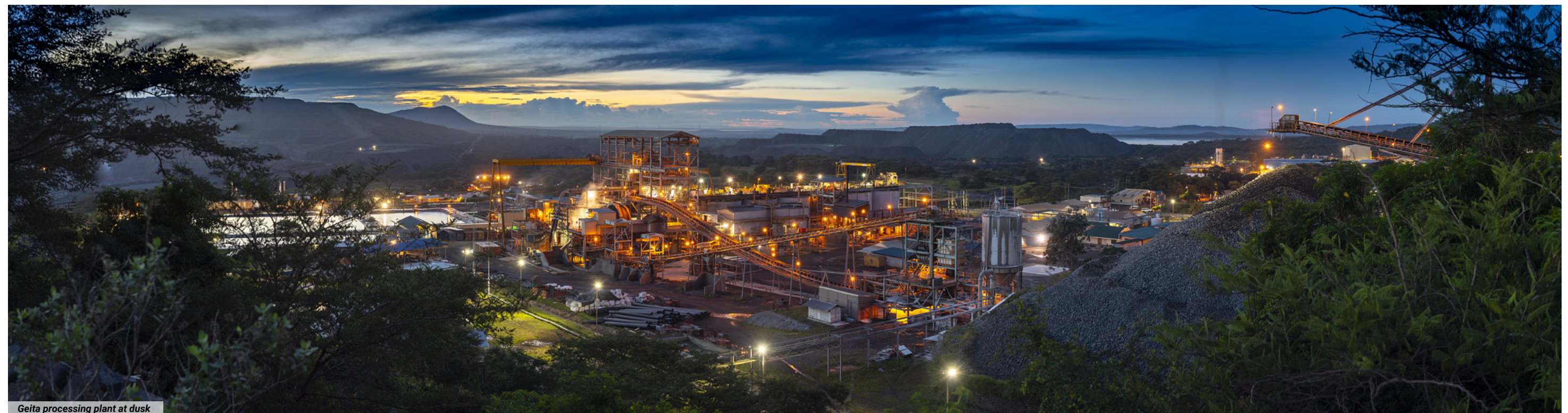
Geita processing plant at dusk
