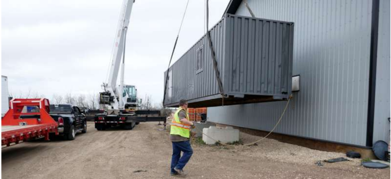
Installing AOS on-site.
