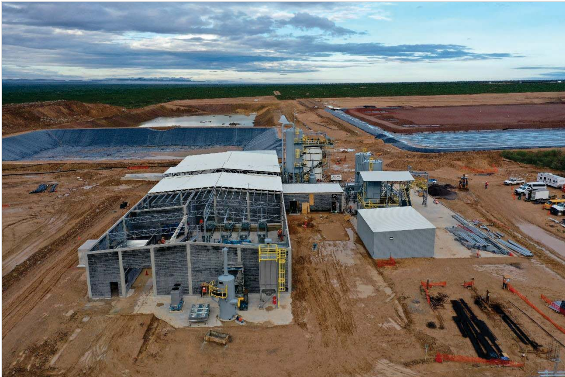
Figure 2: Merrill-Crowe Plant (front centre), Pregnant Pond (back left), Heap Leach Pad (back right)
