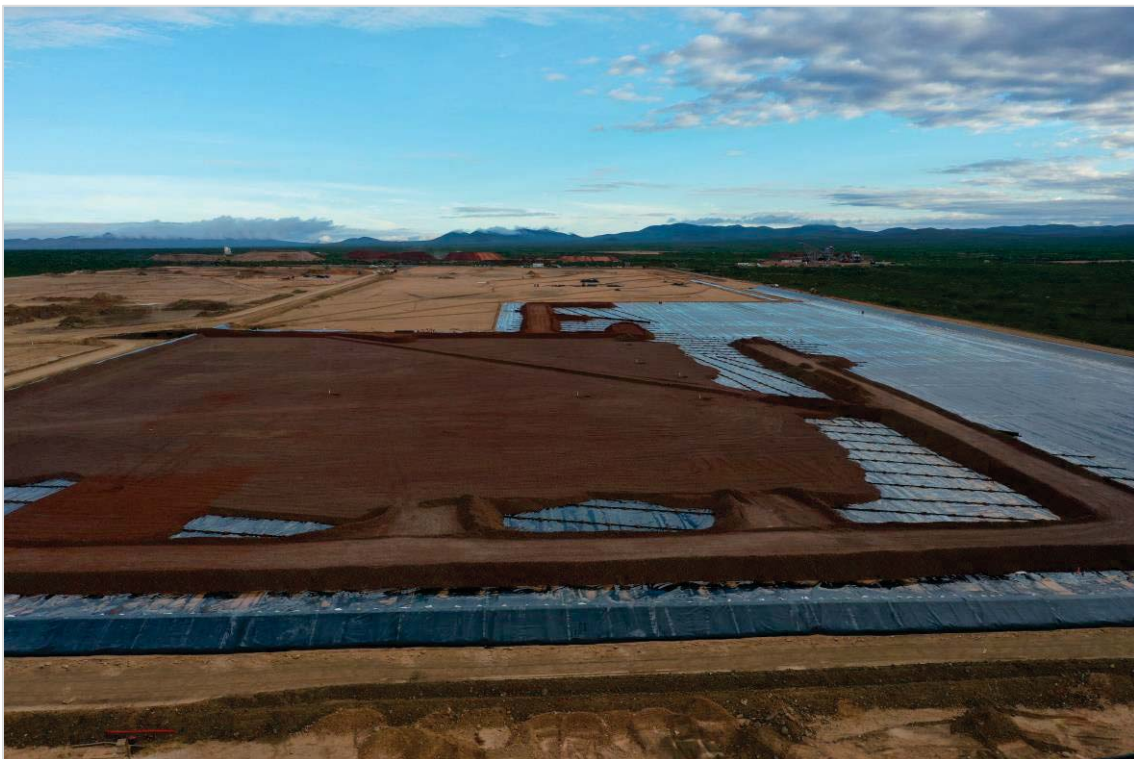
Figure 3: Heap Leach Pad (with placement of overliner material)
