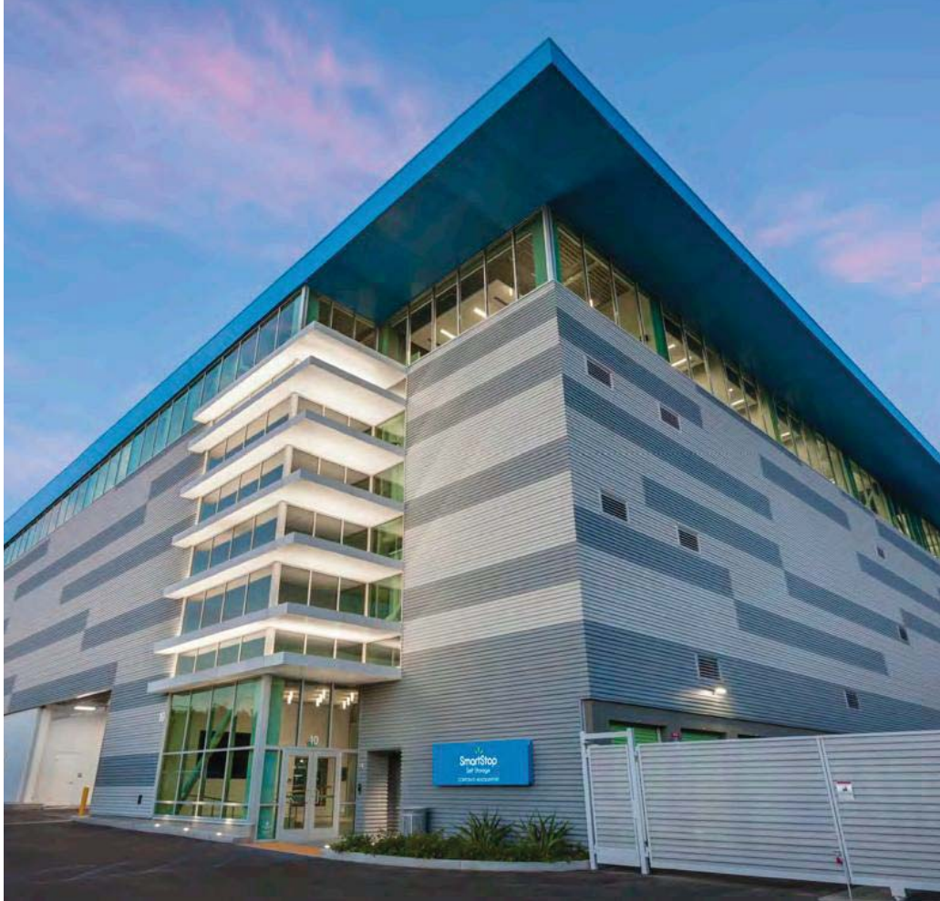
SmartStop Self Storage Corporate Headquarters - 10 Terrace Road, Ladera Ranch, California
