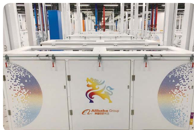
▲ Alibaba Cloud develops a unique “soaking server” cooling system that can save energy compared to traditional mechanical cooling.
