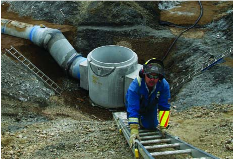
Industrial work at Suncor Energy's Millennium Naptha Unit project
