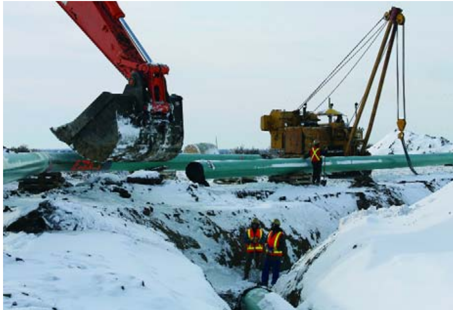
Pipeline installation for Lloydminster to Wainwright Mainline Loop Project
