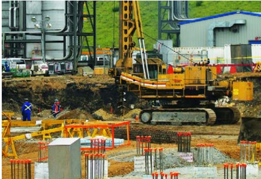
Piling work at Suncor Energy's Millennium Naptha Unit project
