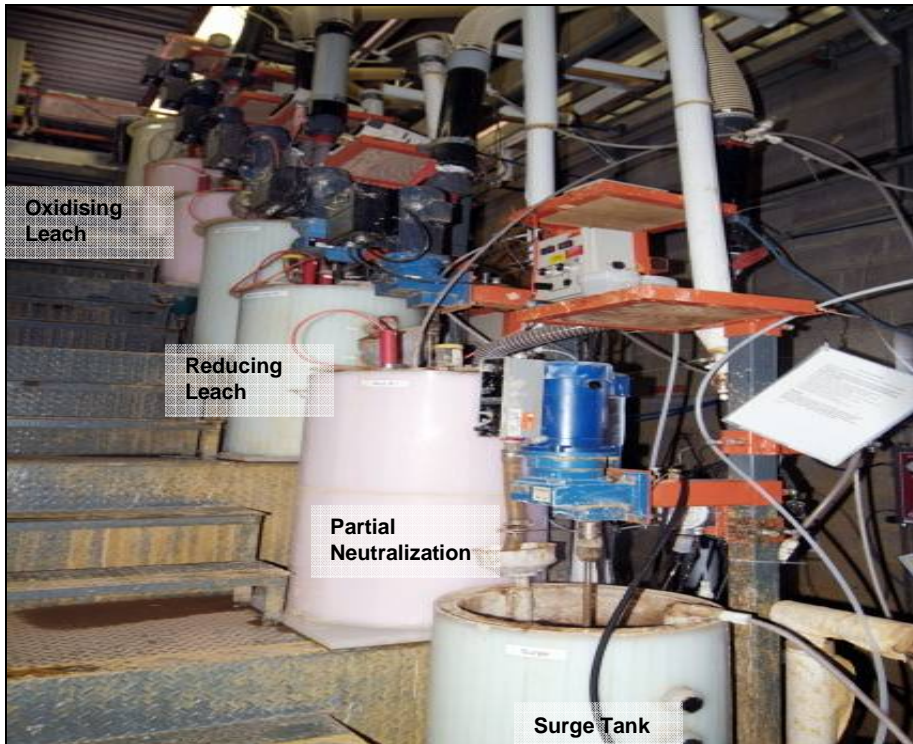
Photo 1 Overview of the Leach Circuit.
