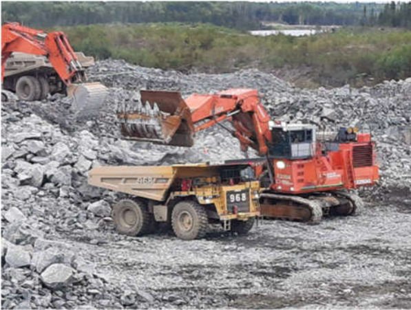
Earthworks – Loading and Hauling
