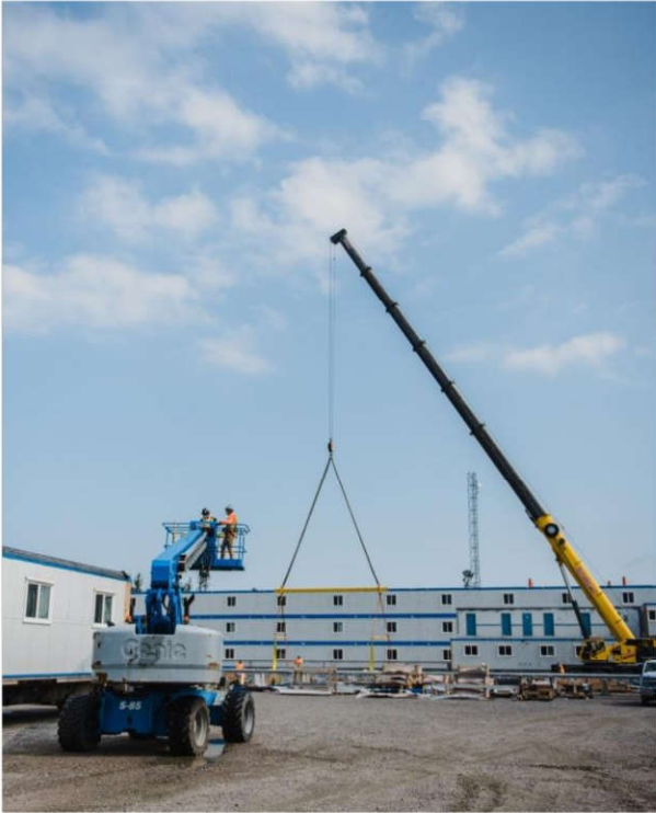
Permanent Camp Construction
