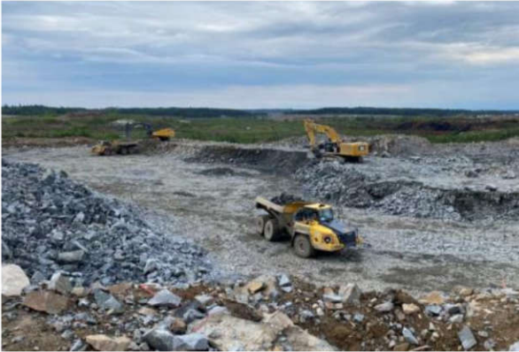
Earthworks – Loading and Hauling
