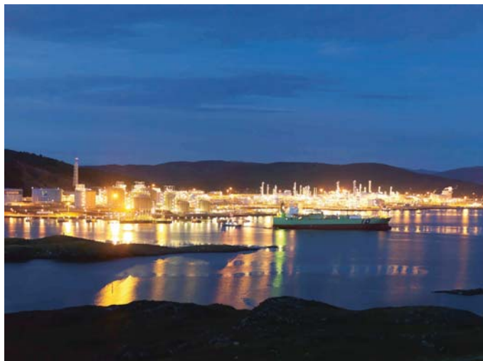
Kårstø. Kårstø is currently preparing for the future with the ongoing KEP.
