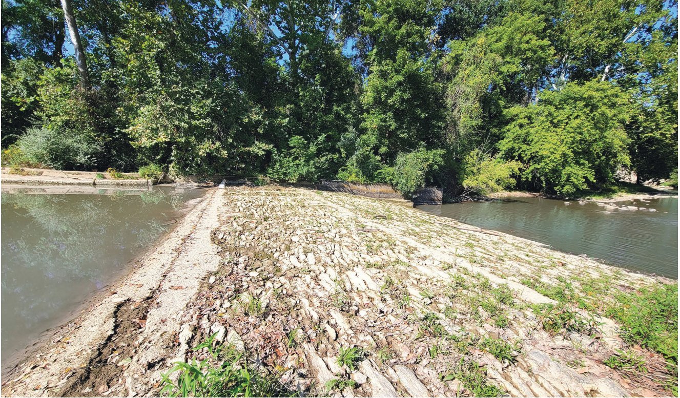
South Branch Codorus Creek at Brillhart Pumping Station, summer 2023.
