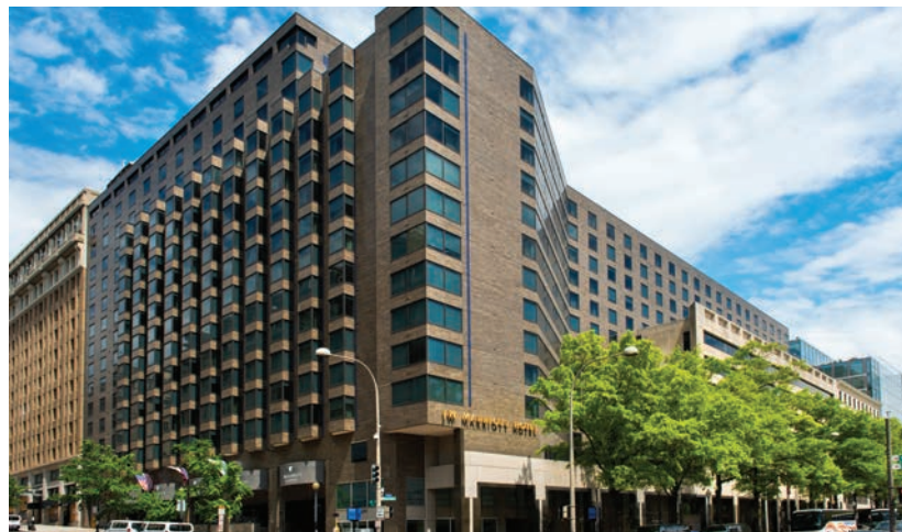
JW MARRIOTT WASHINGTON, DC (Achieved LEED EBOM Gold certification in 2022)
