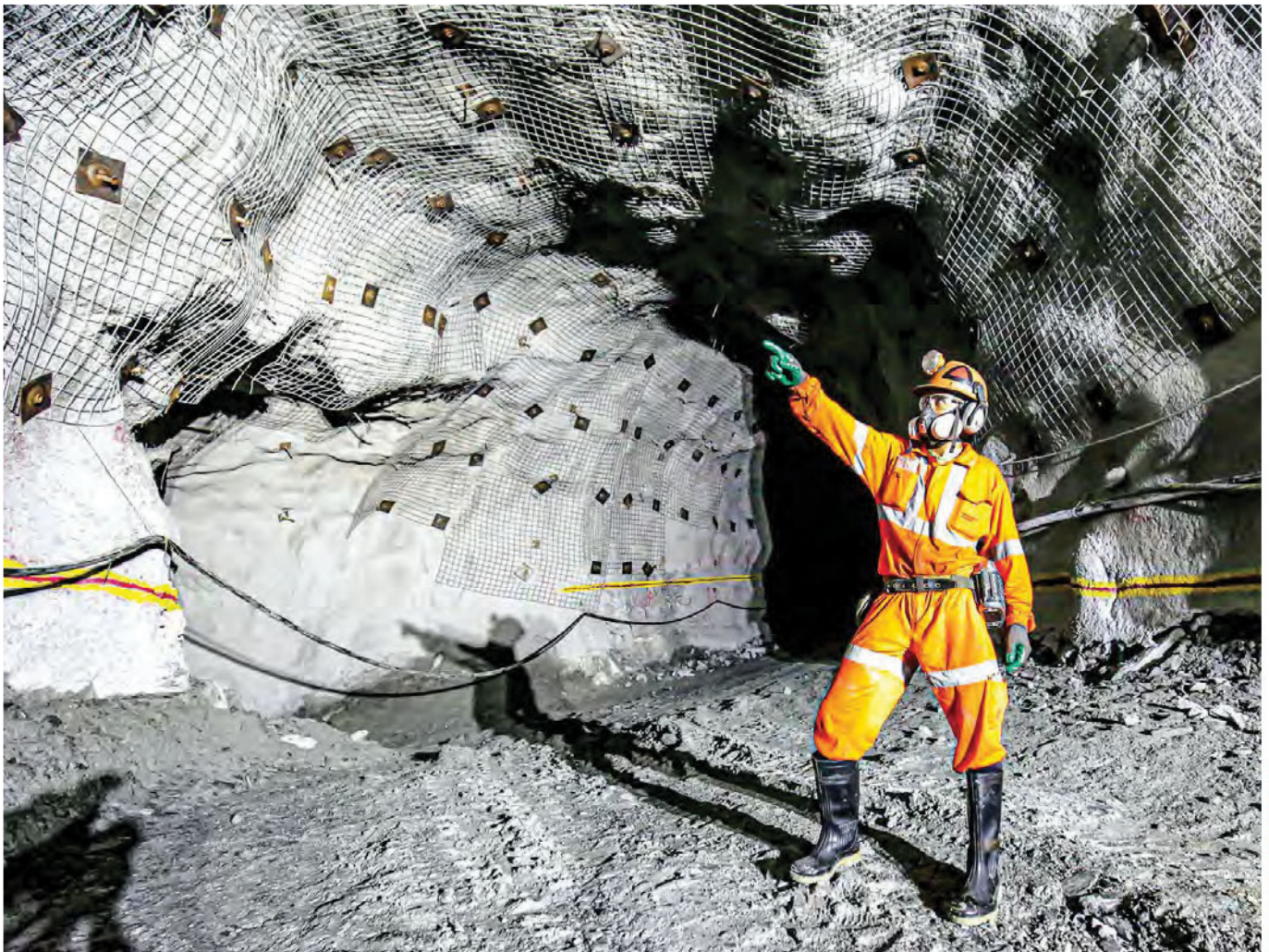
Roof support at the Cuiabá declines
