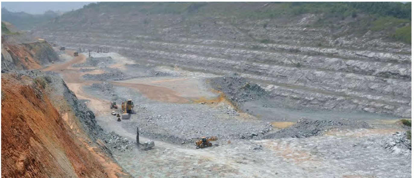
Open pit mining at Blocks 7 and 8 - Cut 2, at Iduapriem
