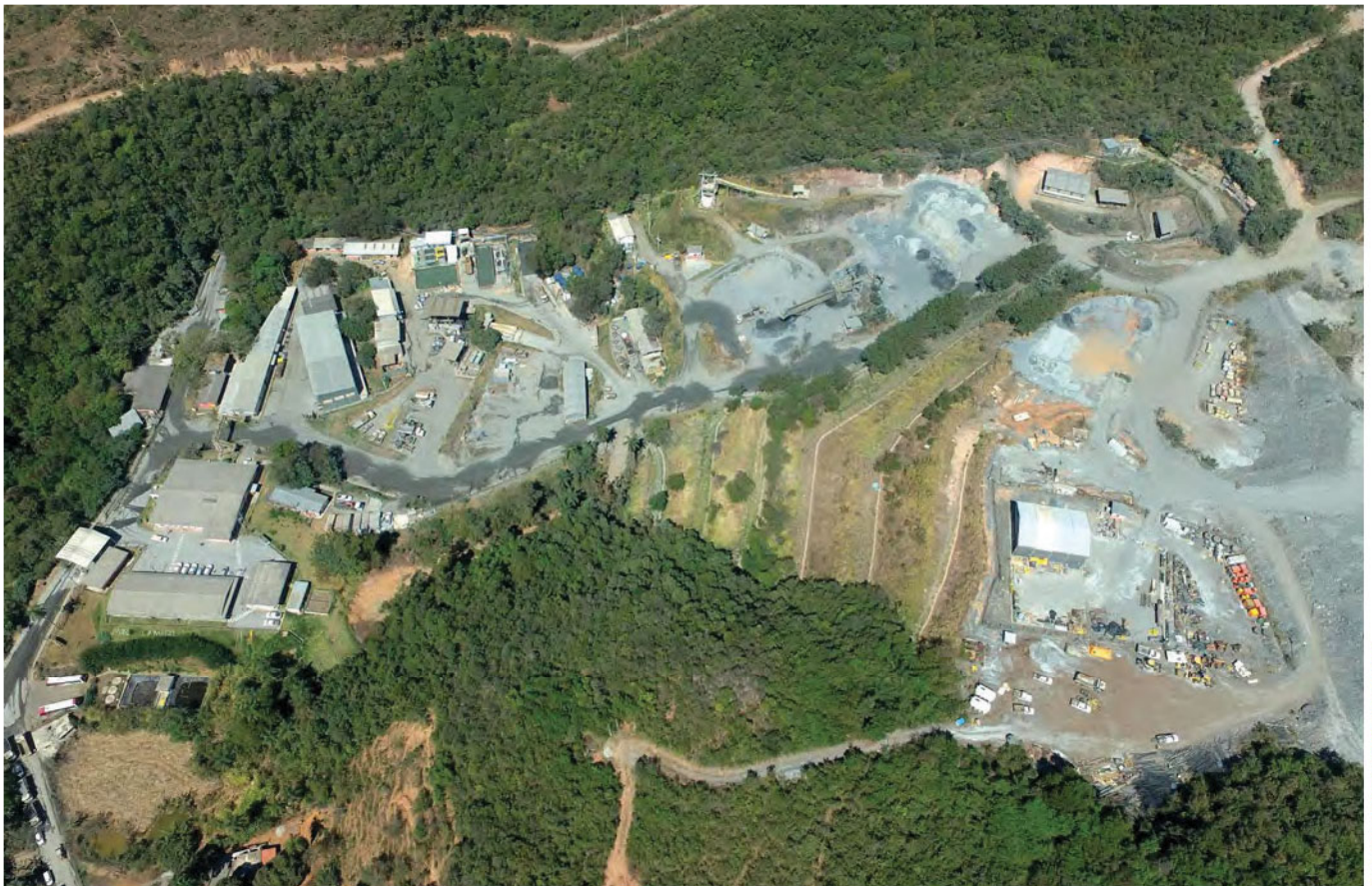
Aerial view of the infrastructure at Lamego
