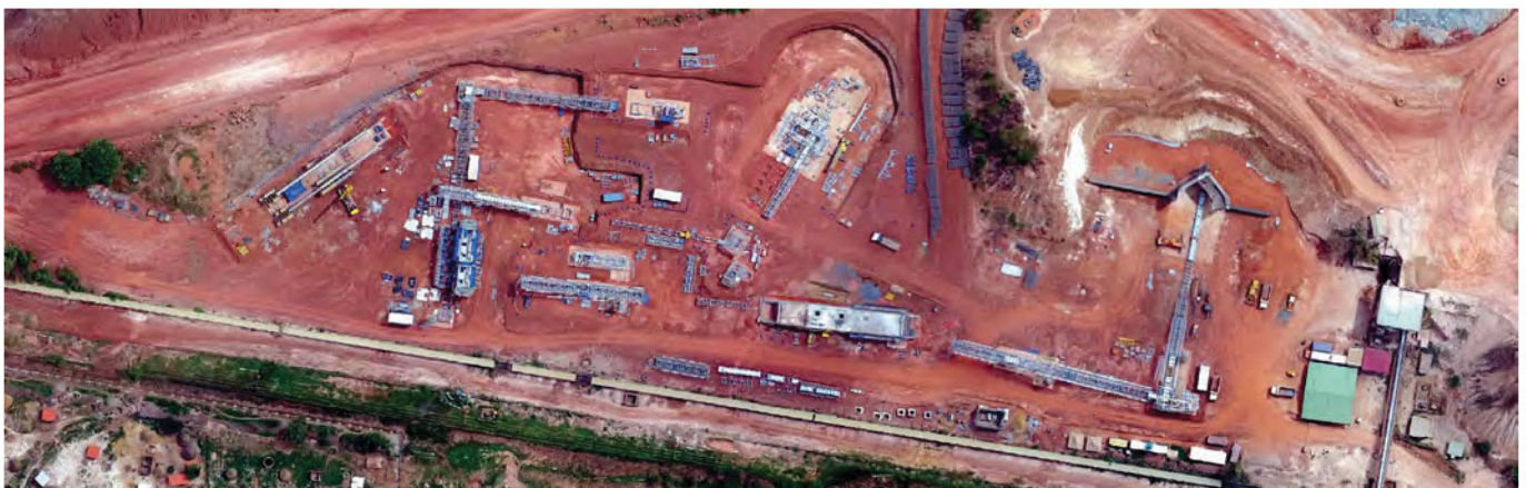
Aerial view of the Siguirí crusher
