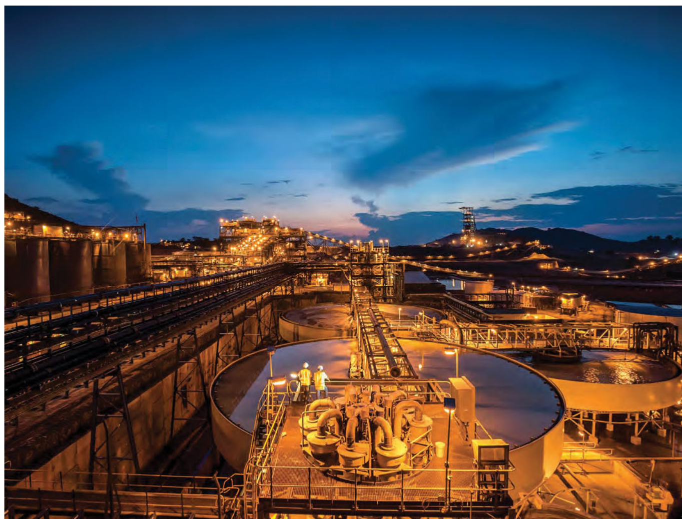
Kibali processing plant at night
