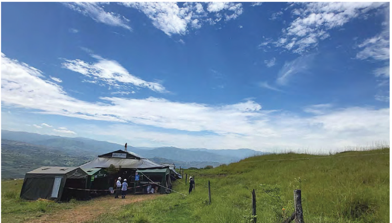
Geotechnical drilling platform at Quebradona
