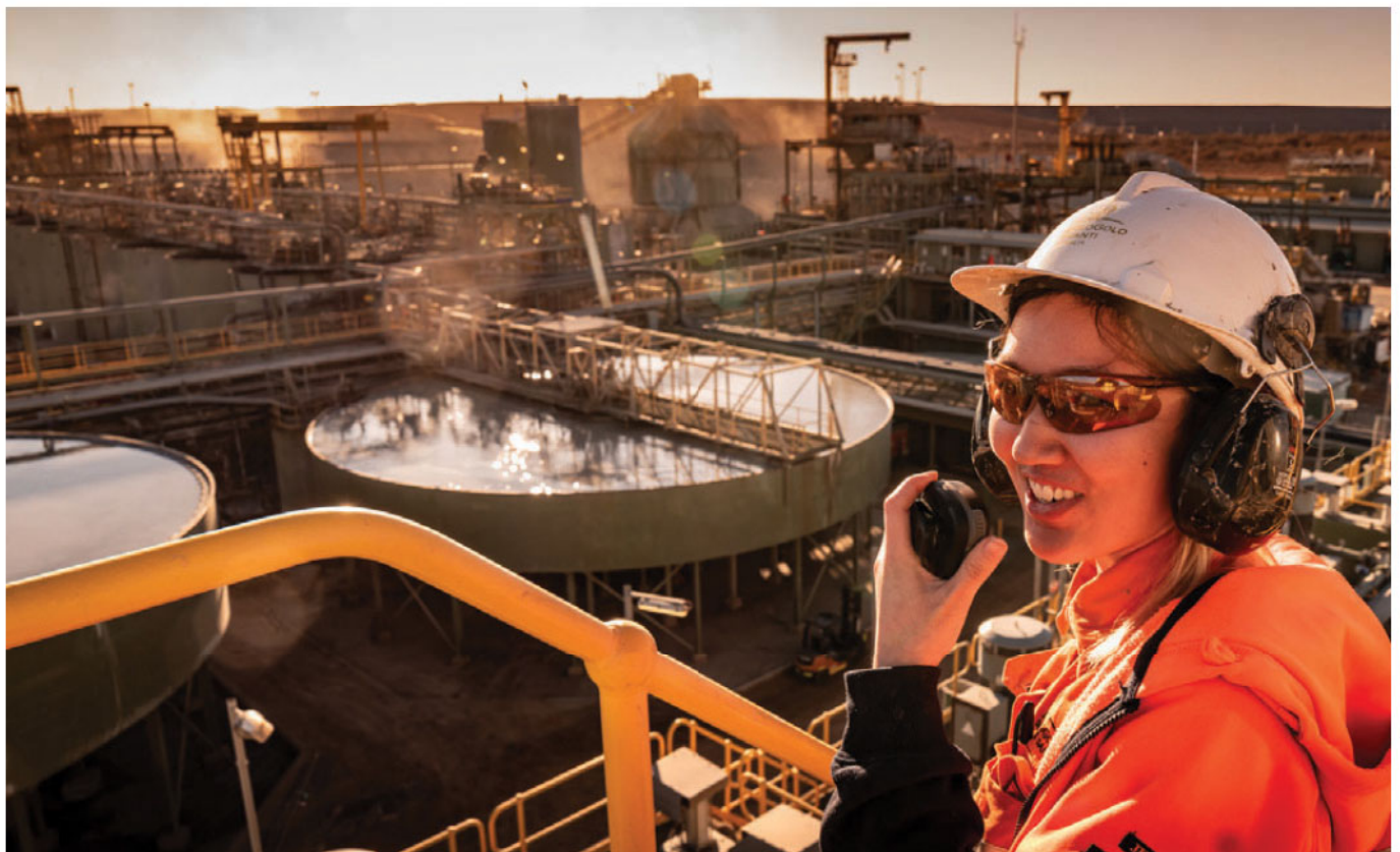
An employee overseeing the thickener tanks
