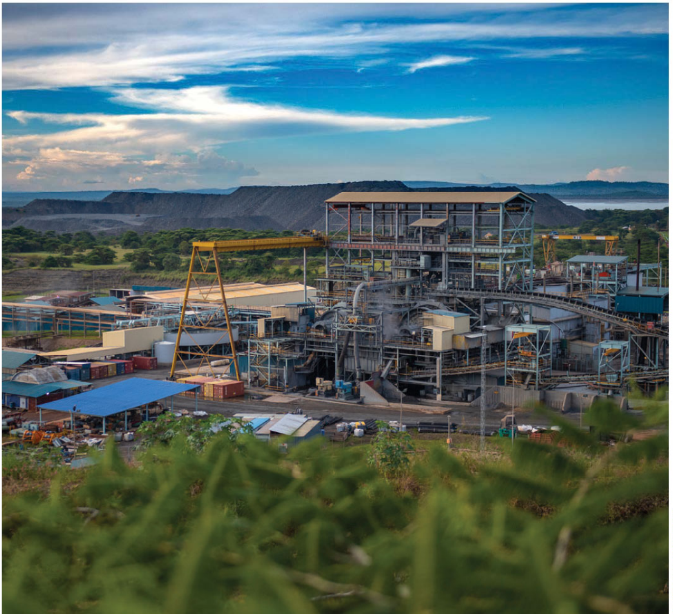
View of the processing plant at Geita
