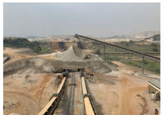
Overlooking the crushing circuit
