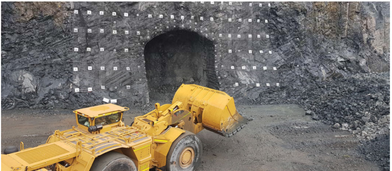
Development of the portal entrance to Nyankanga underground
