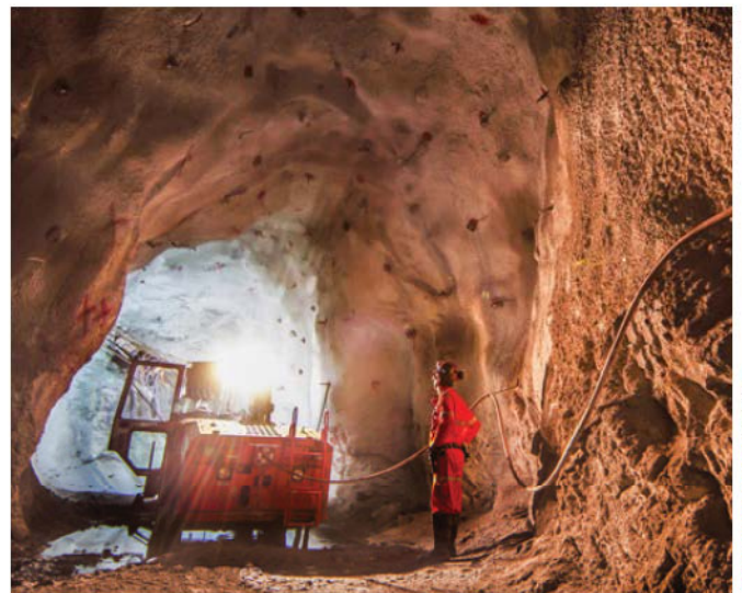
Development drilling underground
