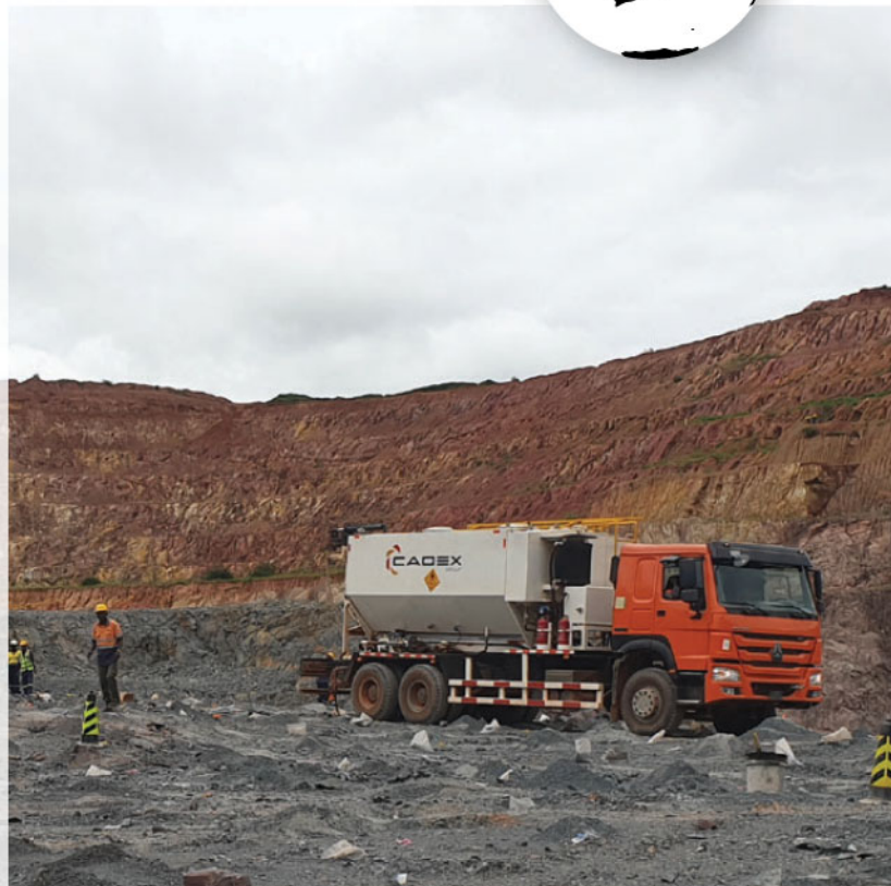
Drilling for padlock blasting at Kami open pit, Siguiri
