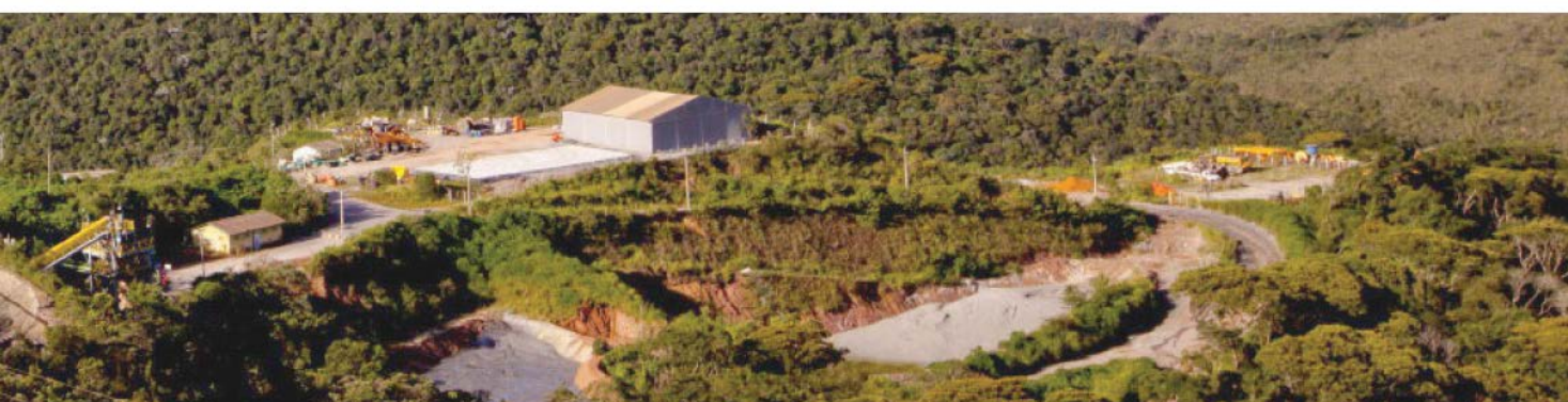
View over the Cuiabá processing plant
