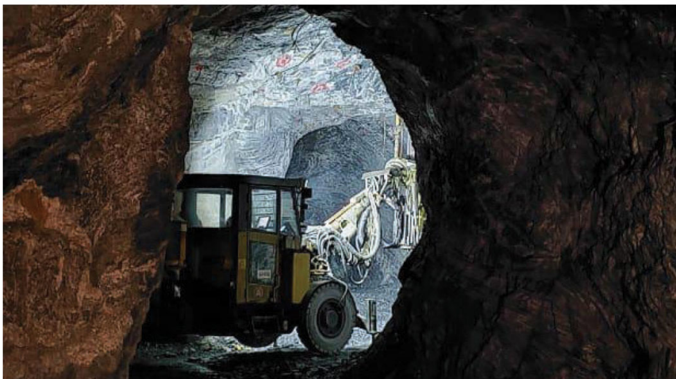
Production drill rig from a distance at Lamago
