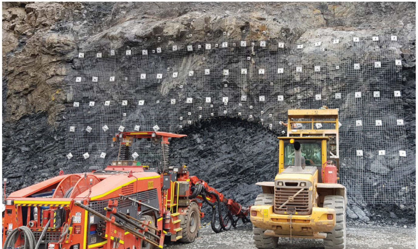
Nyankanga Block 1 portal development
