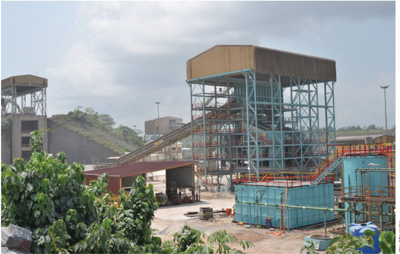
View of the crusher
