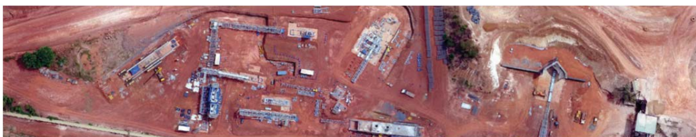
Aerial overview of the Siguiiri crushing circuit
