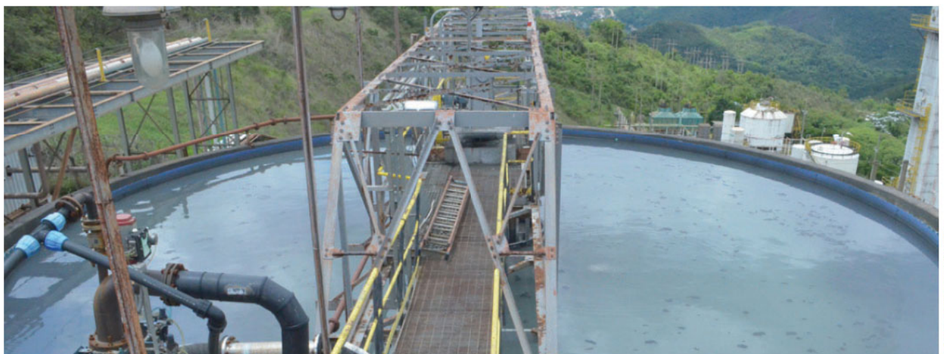
Thickeners at the processing plant
