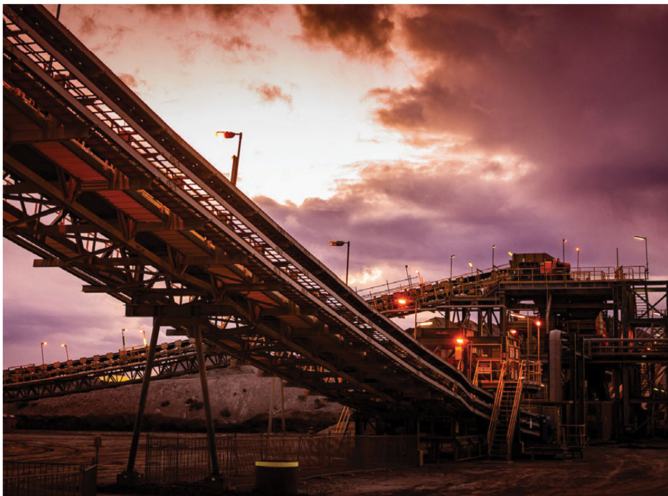
Crushing circuit at sunset
