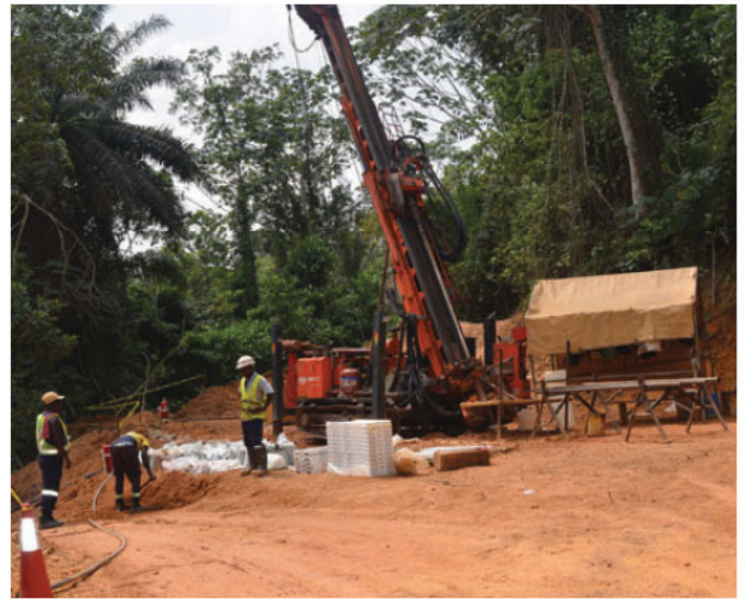
RC exploration drilling
