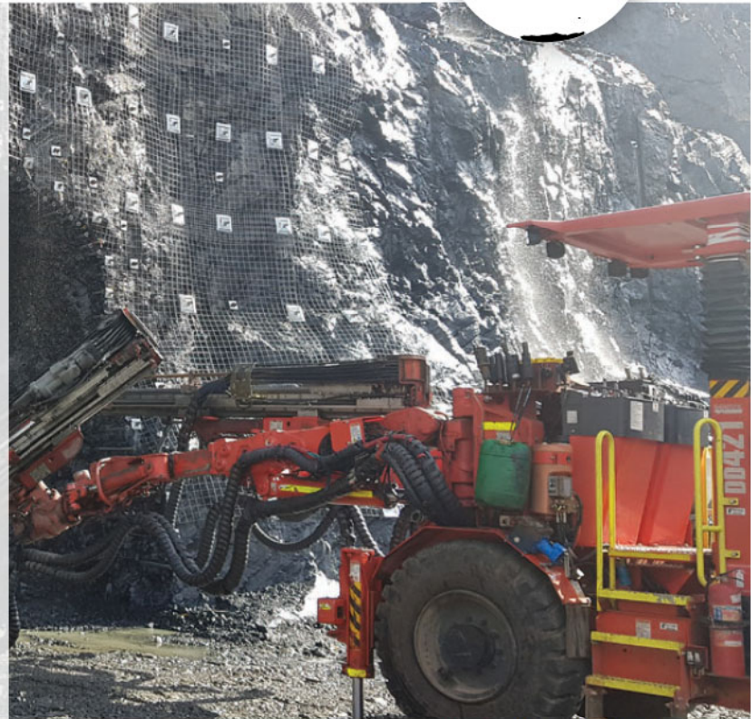
Production drilling at Nyankanga Block 1 portal
