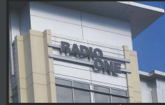
Radio One Headquarters Silver Spring, Maryland
