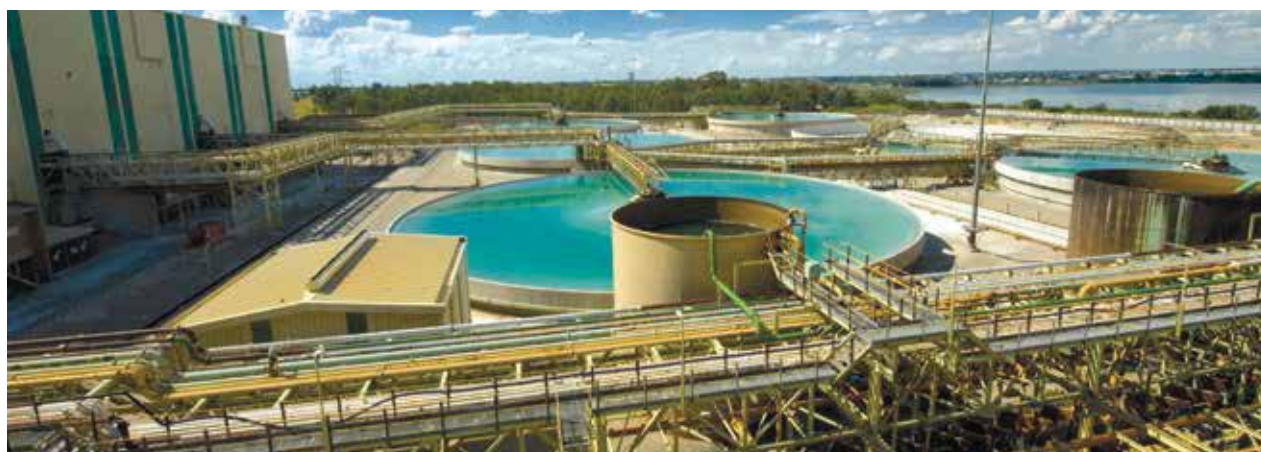
Phoenix tailings retreatment plant
