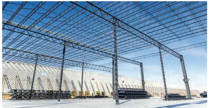
► New Millennium steel joist installation at a jobsite
