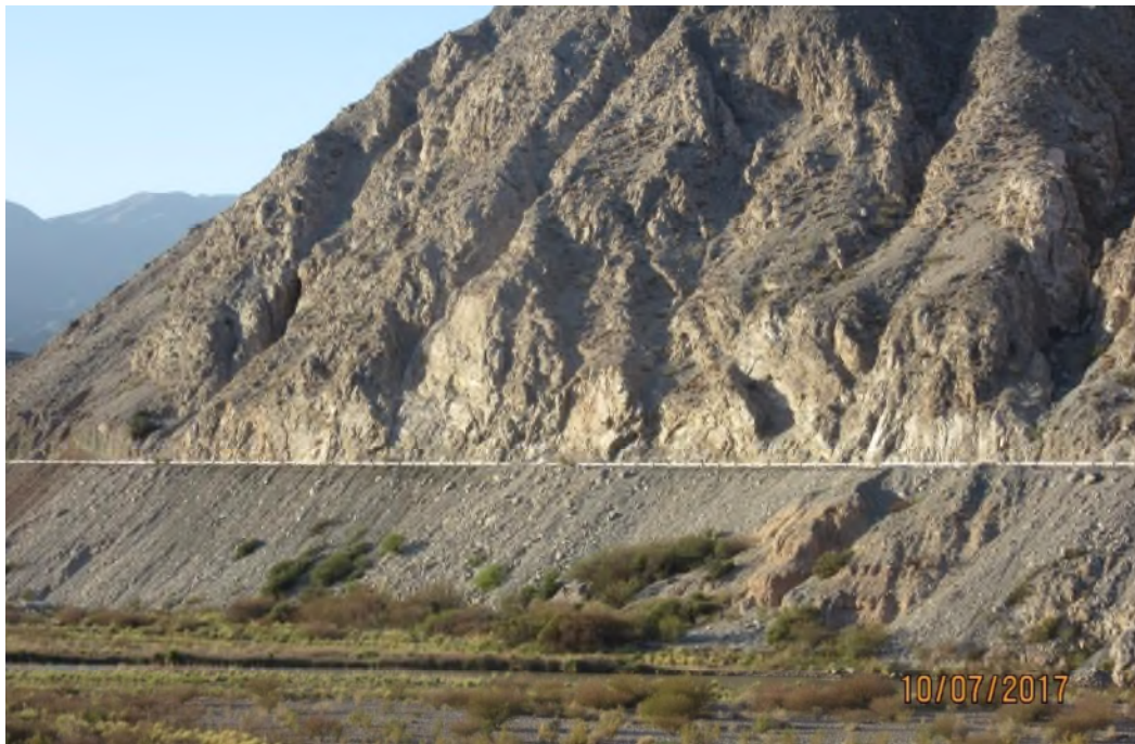
Figure 23-3 A road constructed through the challenging section of the Northern Route would look similar to this road excavated in a very steep rock slope with the road platform well above any potential peak river flow.
