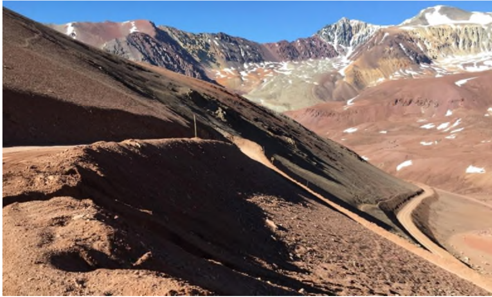
Figure D-1: Recently graded hair pin bends during January 2017 at Tatora Pass on the existing central route to Los Azules, elevation ~4,200 masl.
