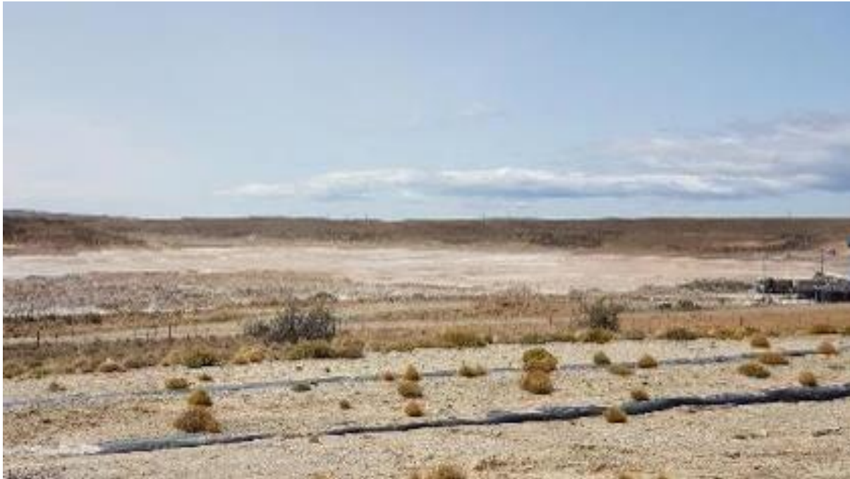
Figure 14-10 – Dry Flotation Tailings Facility #3, January 2020
